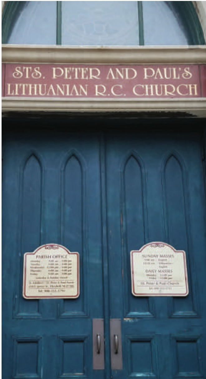
The doors of Sts. Peter and Paul Church in Elizabeth, New Jersey. The church was built in 1910. Above the left door, the Gediminas Pillars (Gedimino stulpai) are still visible. Above the central door, the name of the church is inscribed, indicating that this is a Lithuanian Roman Catholic church, and above the right door, a stylized Vytis, coat of arms of Lithuania is depicted. The mass schedule indicates that Lithuanian/English Mass is held on Sundays at 10:30 a.m. Photo by Rita Janz.
