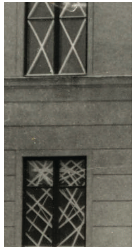
The Martynas Mažvydas National Library building was used by the Red Cross. The windows are "ready" in case of a bombardment.
