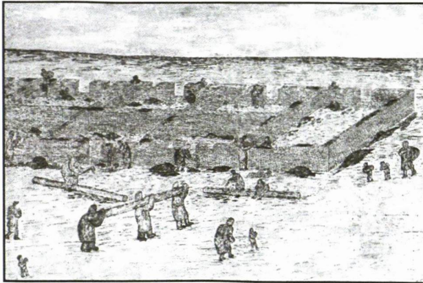
6) - Building the stone barrack. One barrack (100 m x 20 m) was built of bricks using women and children as laborers. They had to lay the bricks on a permafrost ground, filling gaps with moss. During the first blizzard snow was blown in through the door and cracks in the ceiling.
