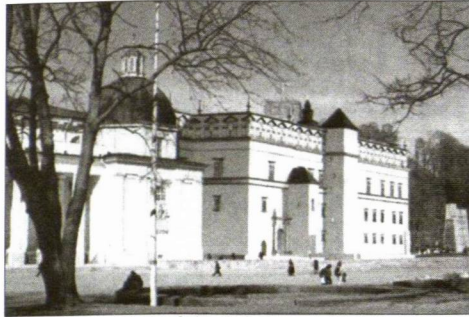
The south wing of the Palace on which the stucco will be applied this summer.
