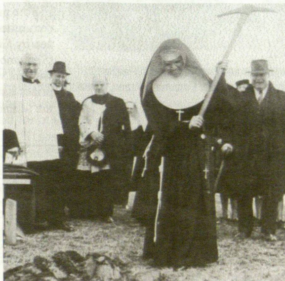
The sisters started to build their motherhouse and ancillary buildings in 1922. They included a school, which is now a daycare center and retreat houses.
