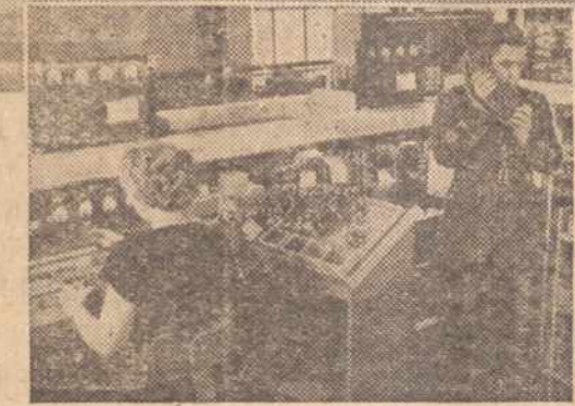
DEFENSE ORDERS demand increased telephone service. To speed production of portable radio military telephones, a new centralized dial system has been installed at the busy Raytheon plant in Waltham, Mass.
