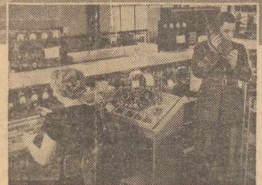
DEFENSE ORDERS demand increased telephone service. To speed production of portable radio military telephones, a new centralized dial system has been installed at the busy Raytheon plant in Waltham, Mass.
