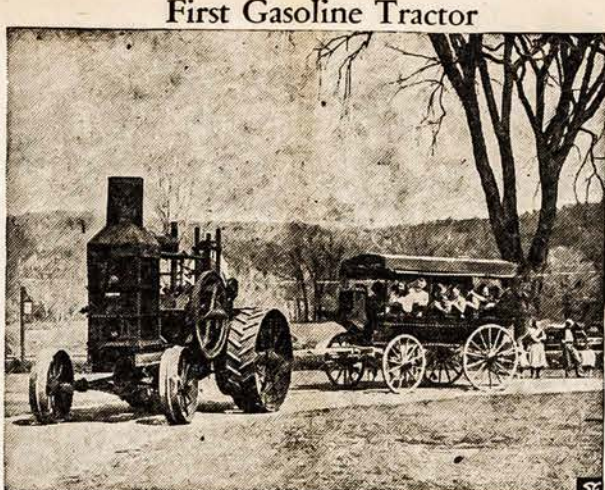
Once around and then to bed was the last "pull" for the first gasoline-driven tractor ever built in the United States. The 19,000 pound agricultural mechanical giant shown above, the Oliver-Hart-Parr, was recently presented to The Farmers' Museum of Cooperstown, New York. Built in the winter of 1902-03 by Hart and Parr at Charles City, Iowa, the tractor has two horizontal cylinders. Gasoline is ignited through a make and break ignition system. Oil circulating through the huge stack acts as a coolant. Since no spark plugs are used, a 1,000 pound flywheel is used to keep pistons in motion during misfiring. After making the "final run" pulling the ancient O-T-E-S-A-G-A Omnibus carrying visiting 4H Club girls... the Oliver-Hart-Parr was assigned an honor spot in the Cooperstown Farmers' Museum Hall of Fame.
