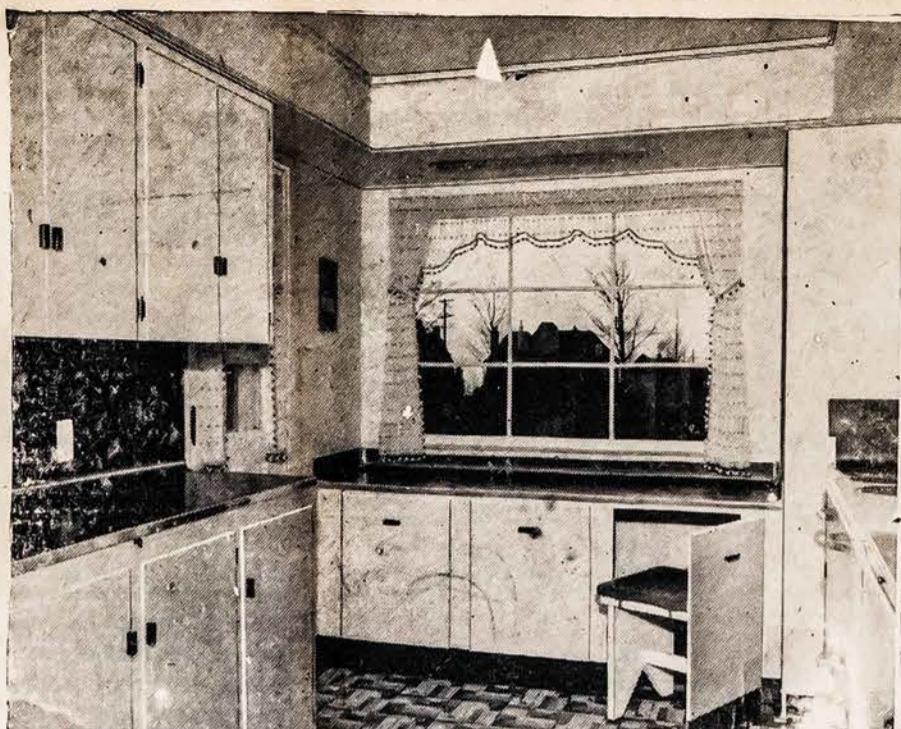
SPACE CONSERVATION! This unusual built-in plywood breakfast bar resembles a cabinet when not in use, requires little space and adds a work surface. A similar installation against any kitchen wall will do much to modernize the room.
